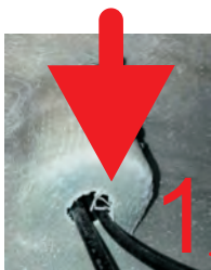
Pass wires from light box into cabinet
